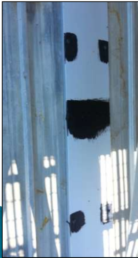
1. RTT Sealant applied to joints and bolt heads
