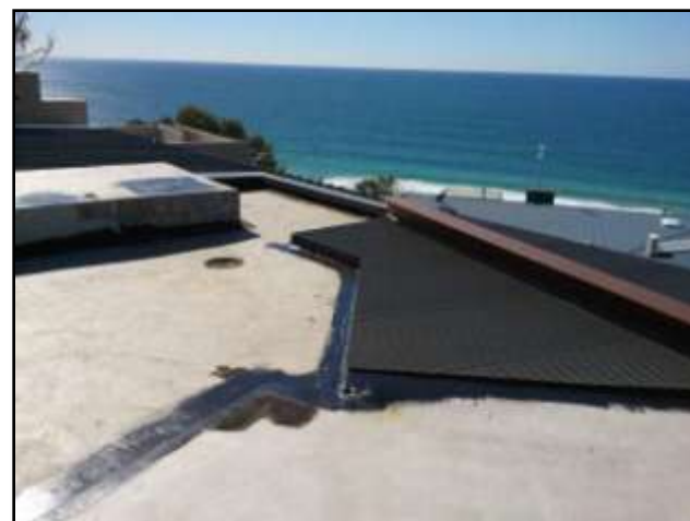
RTT Sealant brush/roller applied
