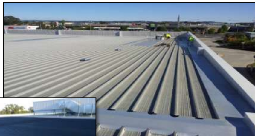
Leaking areas requiring sealing
