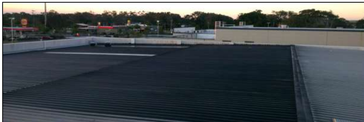
2. RTT Sealant applied to entire area
