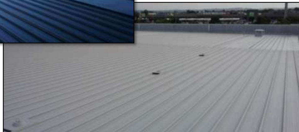
RTT Sealant + Top coat applied to roof to prevent corrosion
