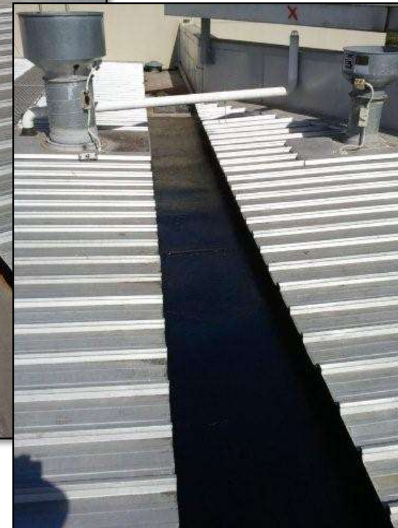
RTT Sealant applied to entire gutter to prevent corrosion
