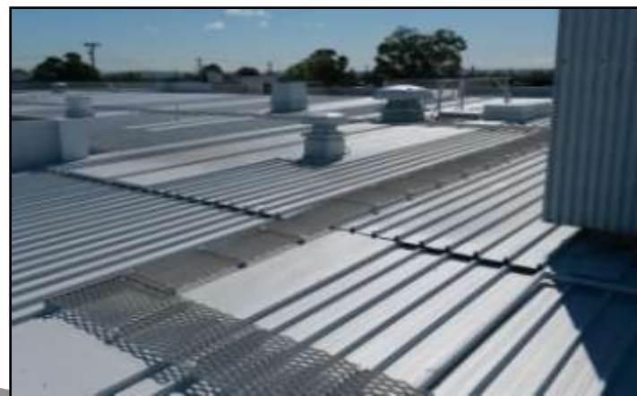
RTT Sealant + Top Coat spray applied
