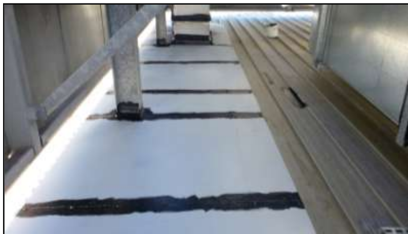
1. RTT Sealant applied to joins and corners
