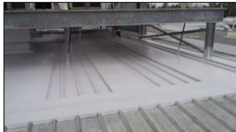
3. Coloured top coat applied to RTT Sealant
