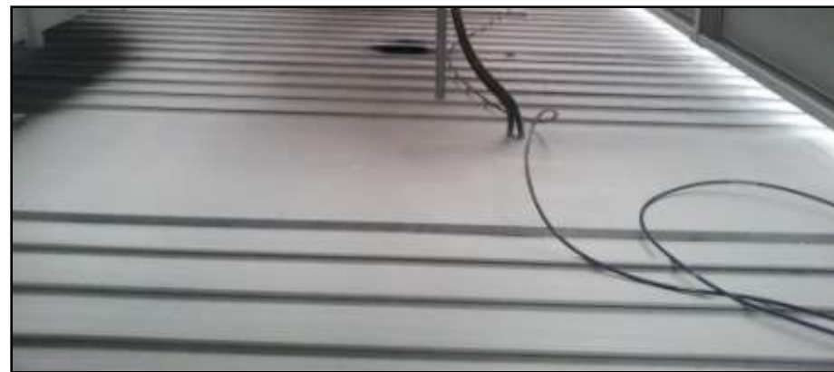
3. Coloured top coat applied to RTT Sealant
